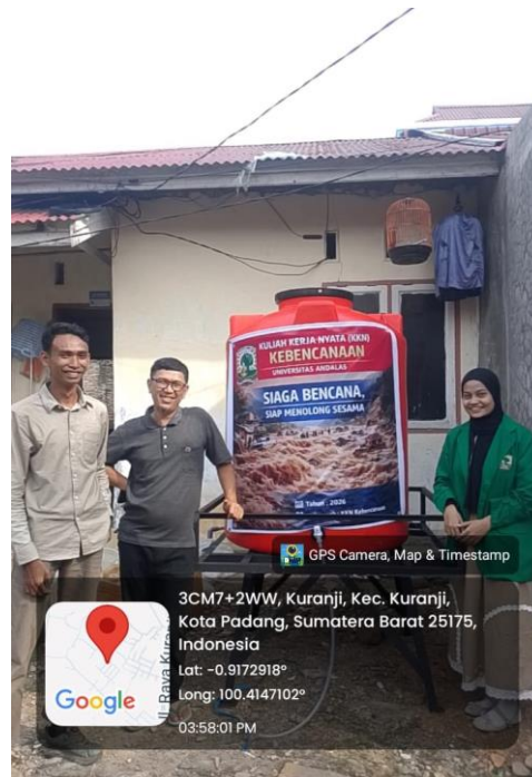
Figure 1. Installation of clean water storage tanks in residential areas to improve water accessibility
