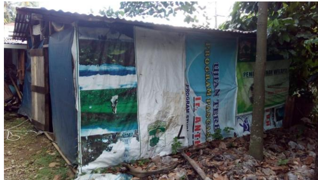
Figure 3. Kumbung before being repaired
