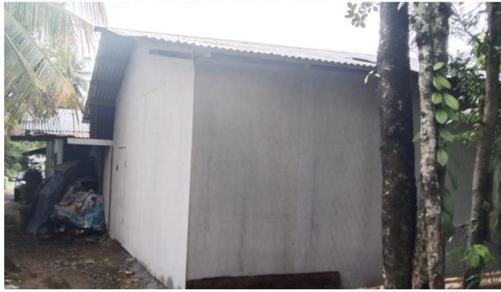
Figure 7. Kumbung after completion of the repair phase
