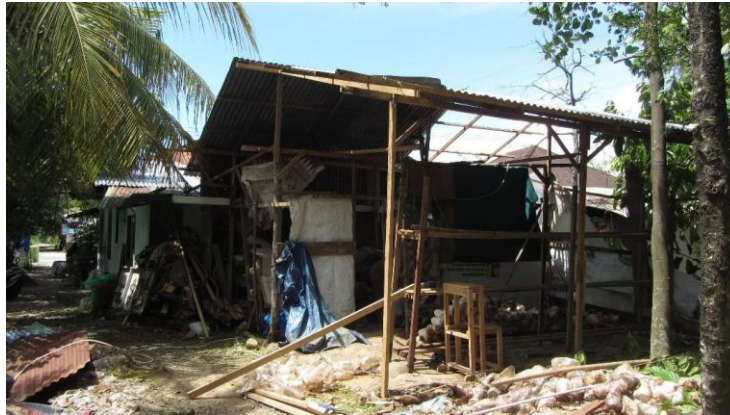
Figure 6. Kumbung under repair
